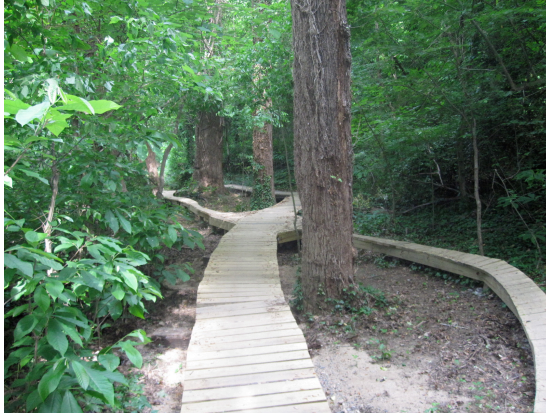
Figure 12: Technical Trail Feature Boardwalk
